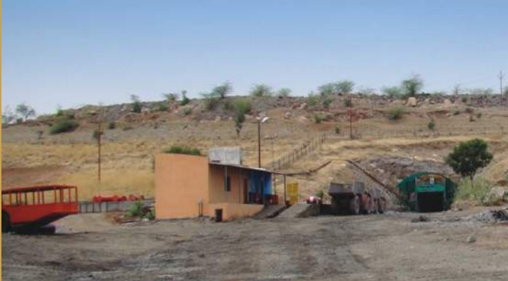
Sindesar Khurd Mine main entrance
