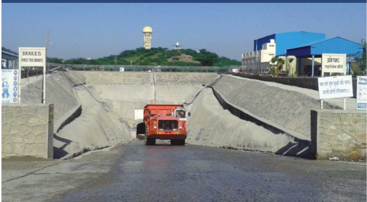
Kayad Mine Portal
