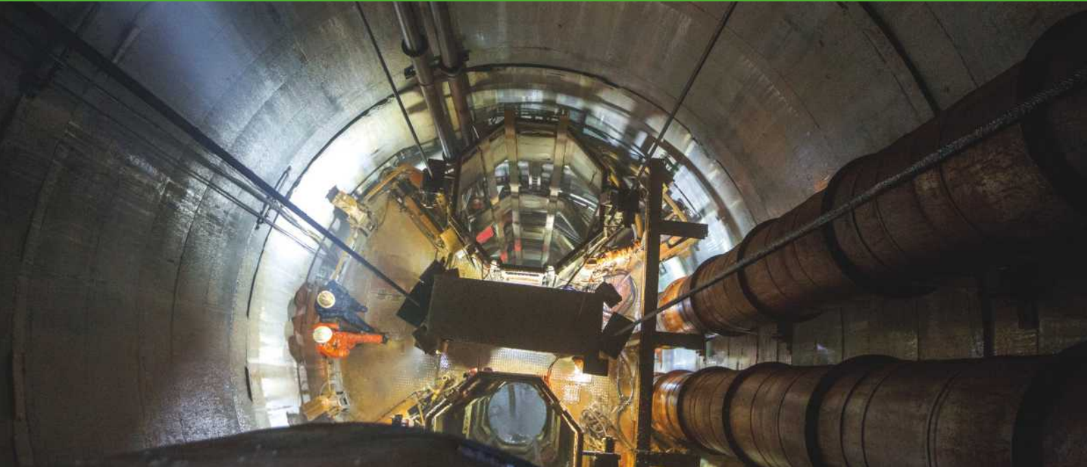
Underground Shaft at Rampura Agucha Mine
